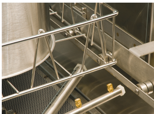
Rollers make getting large racks in and out of the pot washer easier.
