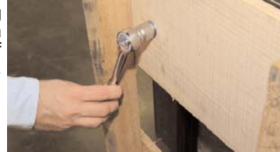
Removing skid from bottom of cabinet.
