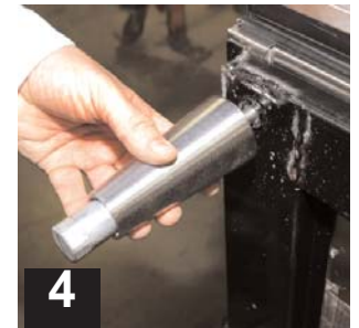
4 Thread leg into cabinet bottom frame rail.
